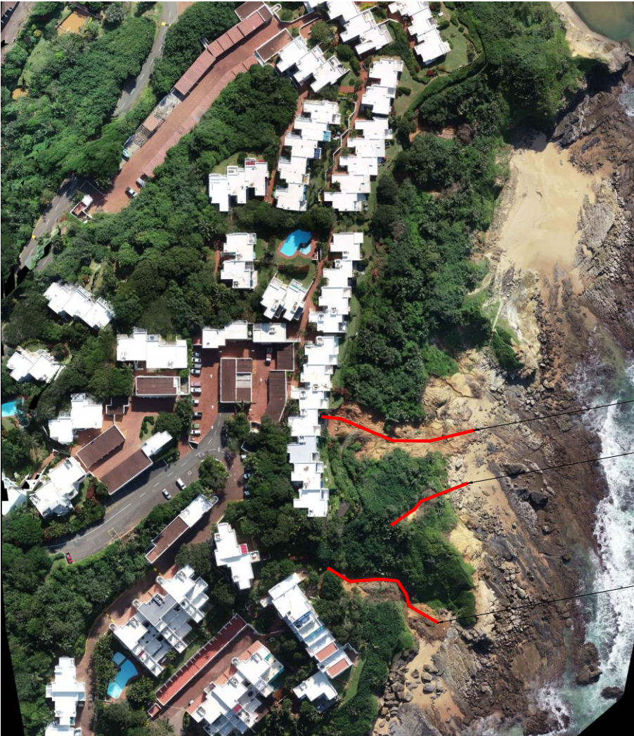
COLLAPSED AREAS AERIAL VIEW
