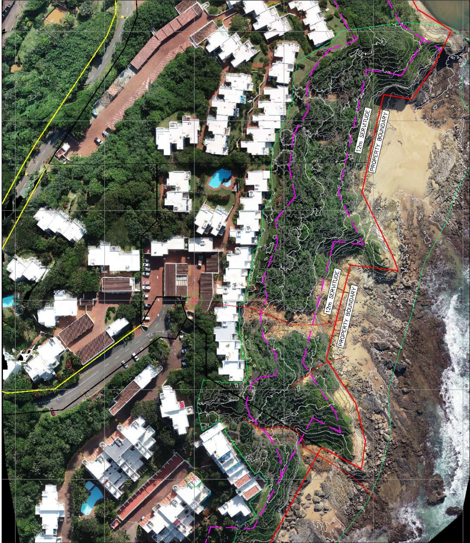
COLLAPSED AREAS AERIAL VIEW
